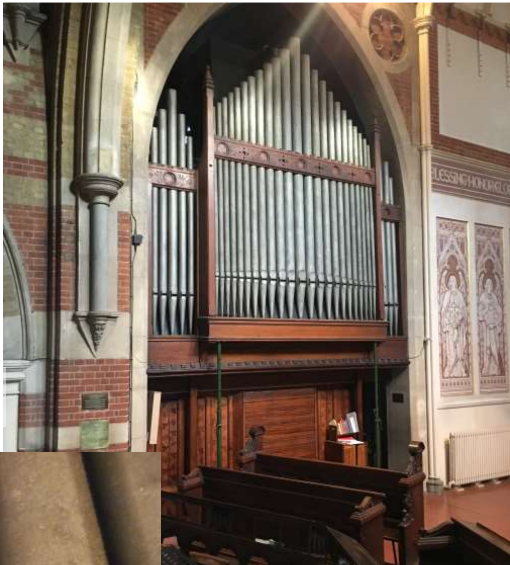
↑ South Case Green props are supporting the "Tip Block"
