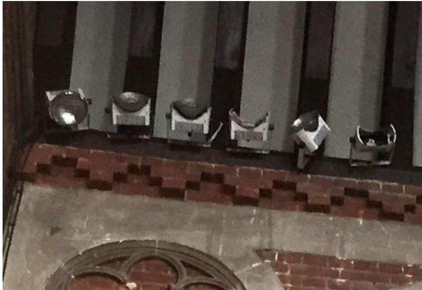
Existing lighting units.
